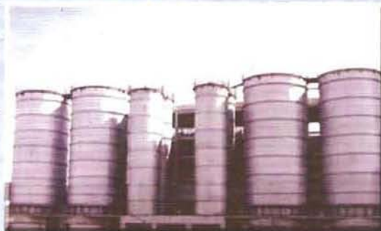
STORAGE TANK AND SILO
