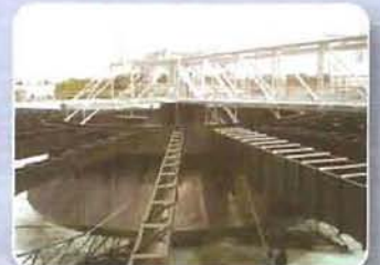
CLARIFIER MECHANISM
